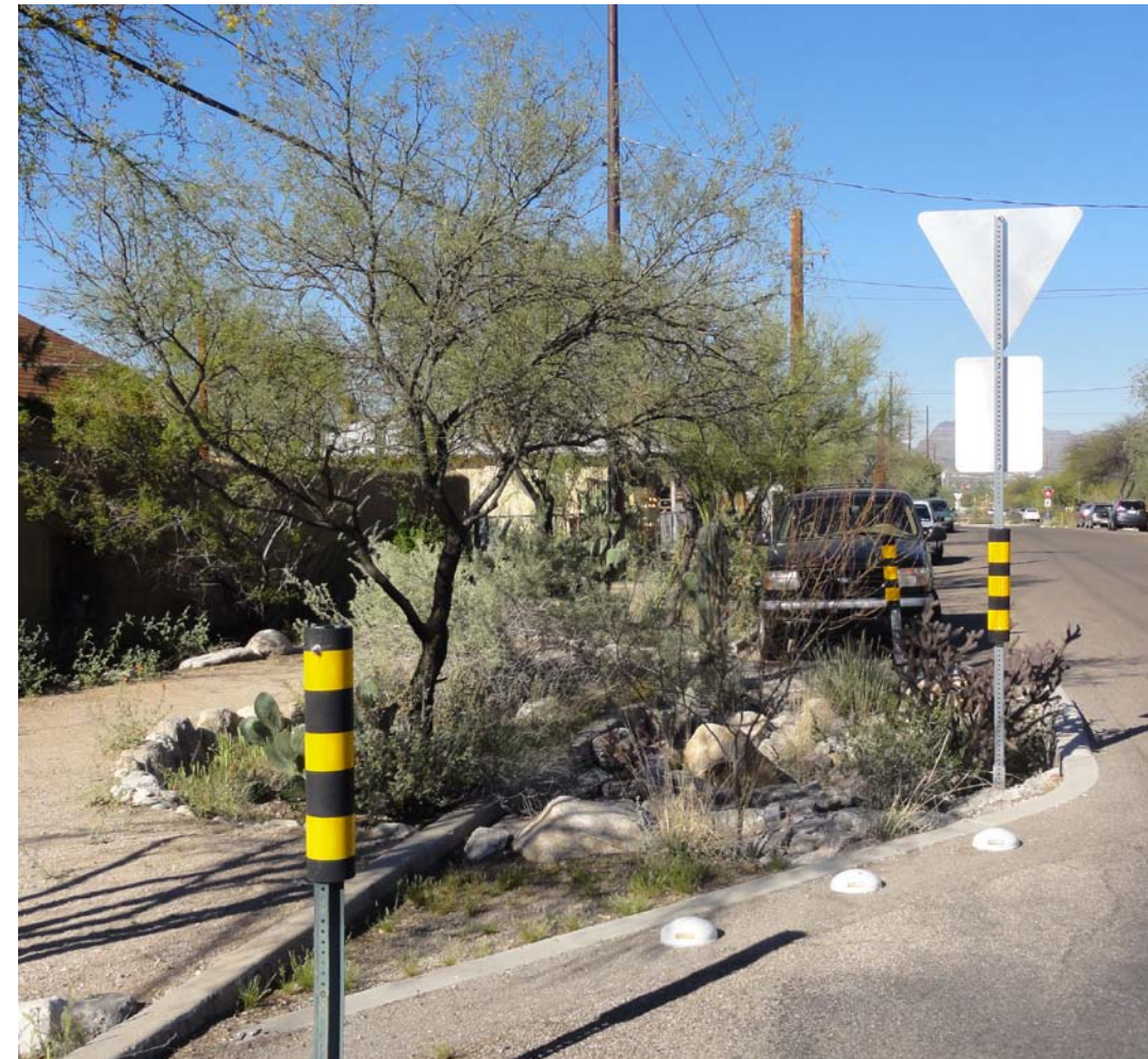
STORMWATER HARVESTING BASIN, TUCSON
